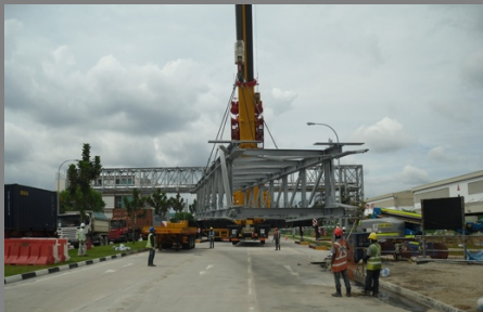
Pipe Bridge installation @ Banyan Place
