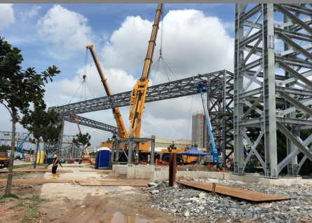
Pipe Bridge installation @ Banyan Place
